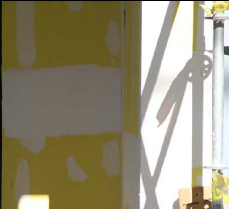
Tape & Float to Create Smooth Surface
